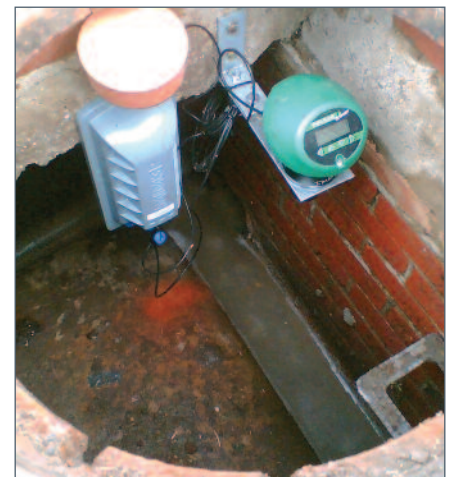
IMP MONITORING IN A CSO CHAMBER
