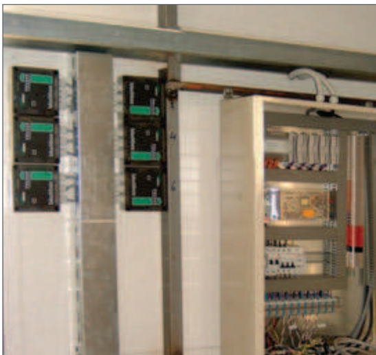
MINERAL OIL TANK LEVEL
